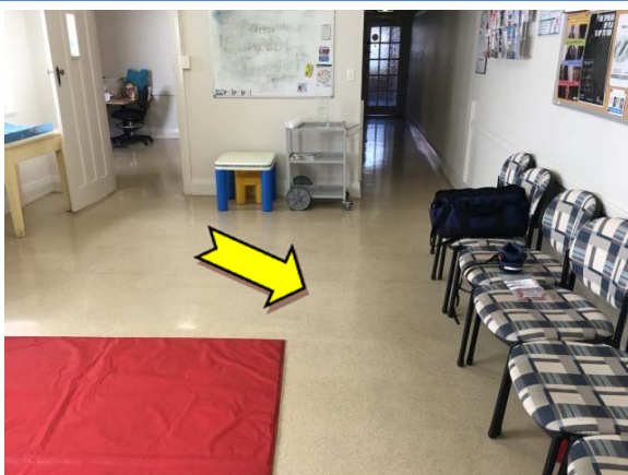
Photo 5. Interior, ground level, throughout, floor – suspected non asbestos-containing vinyl sheeting.
