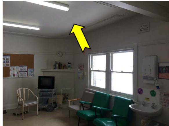
Photo 10. Interior, ground level, throughout, walls and ceiling – suspected lead-containing white upper coloured paint system.
